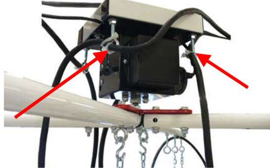
Now tie wrap each wire to the Solar Revolution ARM's at approximately one foot from the end of each ARM. See diagram #5.
